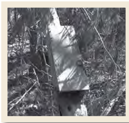
Figure 21. Leaning pole set with use of a cubby box
